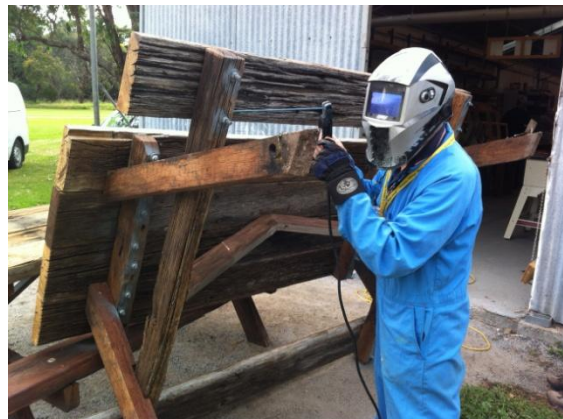
and then Ron welds the nuts, they hopefully will last.
