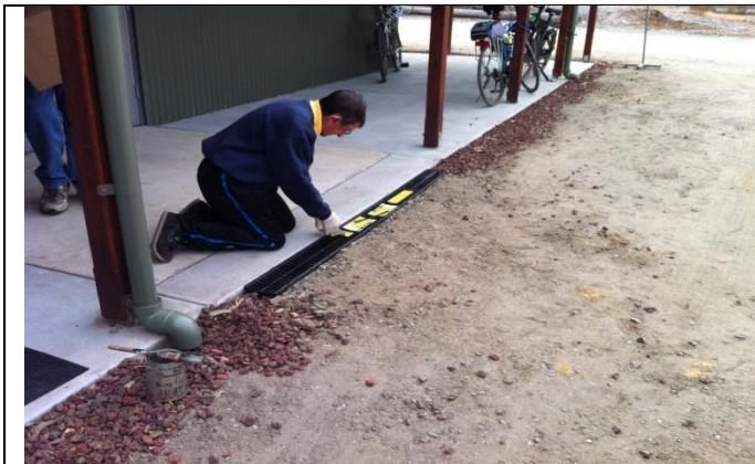
Frank putting the finishing touches onto the perimeter drain for the shed extension.
