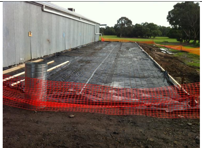
Best news of all ..... the workshop shed extension is underway with the foundation piles having been cast and the concrete slab about to be poured.
