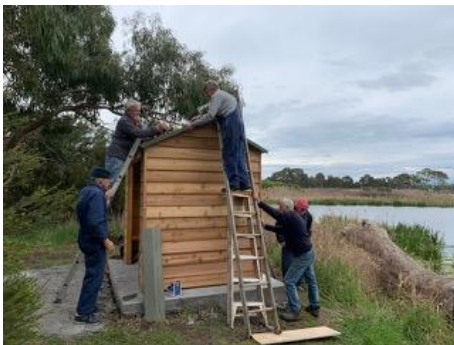
Flashings going on.
