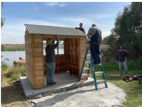
Roof going on the rear wall.
