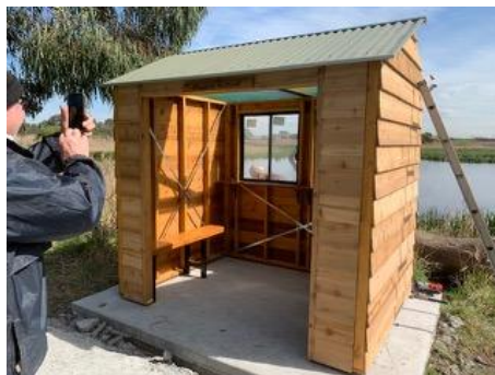
Roof on this side with seats and shelf installed.
